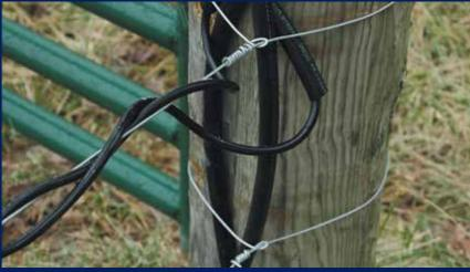
Always use underground cable designed for electric fencing and place it in protective tubing. It is very important to only use underground cable that is designed for electric fence. Never use any product that is intended for residential use. Whenever a cable carrying current is run under the ground, always place it in some type of pipe or conduit that will protect it from future damage. Wires going under gates should be buried to a depth of approximately 1 foot.
