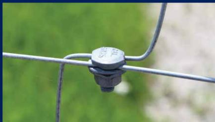
Always connect electrified wires with clamps. Loose connections result in loss of voltage. Connections should NOT be wrapped, but rather clamped together with a high-quality clamp that is designed for high tensile fencing. Never use clamps that are constructed of dissimilar metals. Although economy clamps constructed of cast metal are sometimes available, they often fail upon tightening. Saving a few cents on clamps often leads to exponential headaches in the future.
